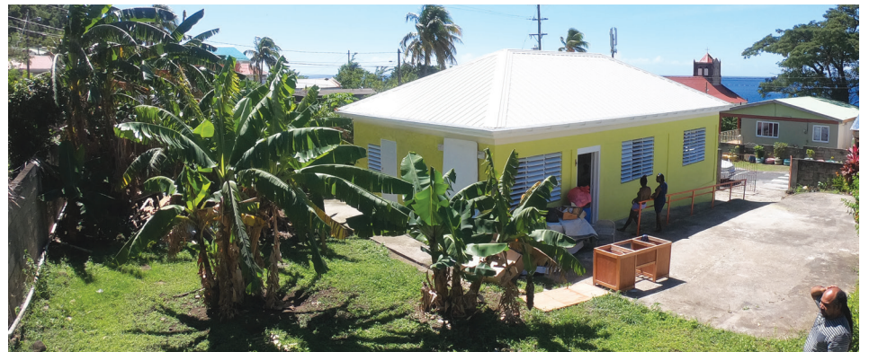
In the aftermath of Hurricane Maria, AmeriCares has rebuilt 11 primary health centers throughout Dominica.
